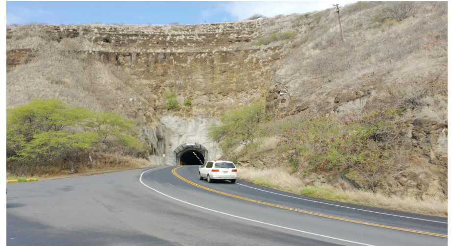
3) Entering Kahala Tunnel
