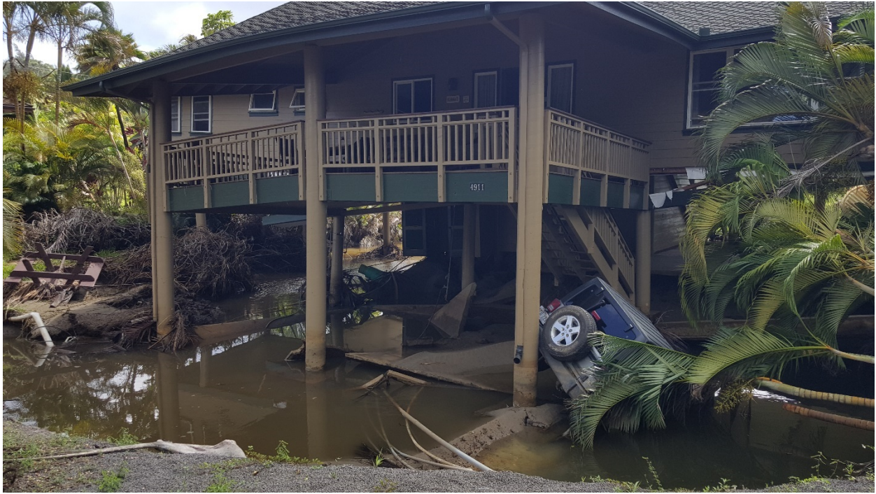
Above: A damaged home and vehicle on Weke Road, Hanalei, Kaua'i.
