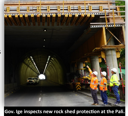
Gov. Ige inspects new rock shed protection at the Pali.
